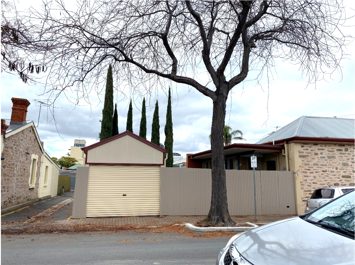
Figure 3.9 – View to subject site and adjacent properties from Collins Street
