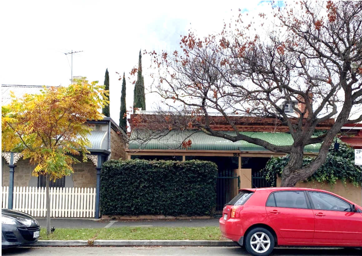
Figure 3.1 – Subject site viewed from southern side of Gilbert Street
